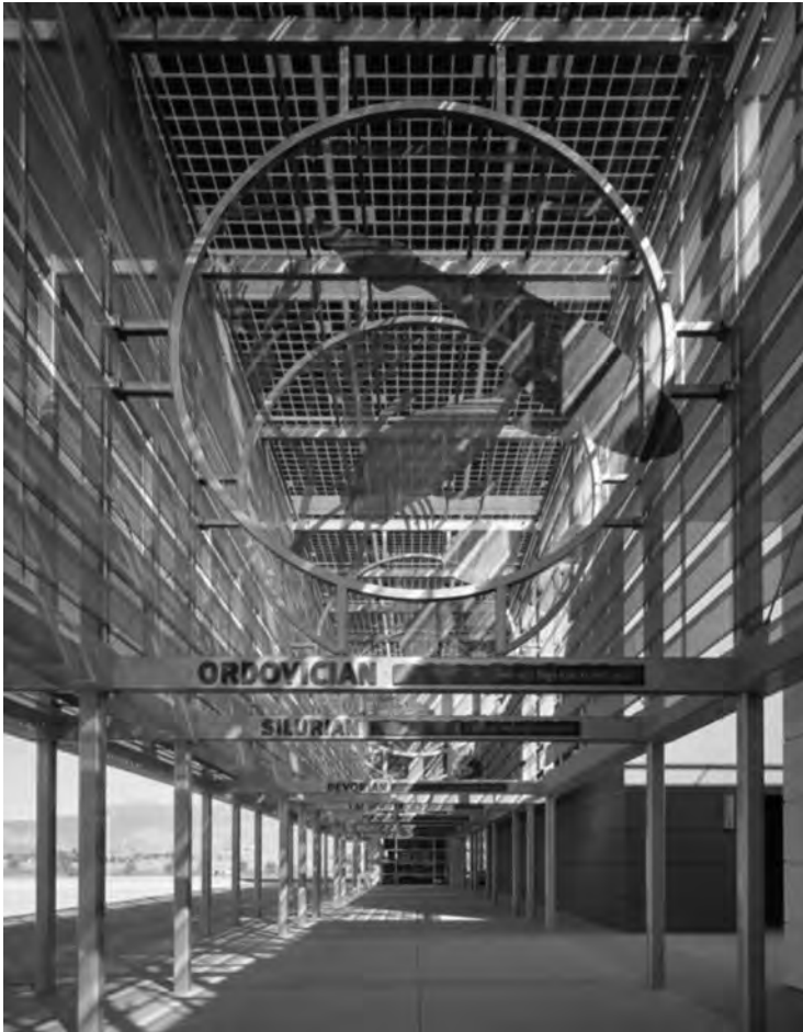
Figure B.31 BIPV solar power logia in Water and Life Museum. Photo courtesy of Fotoworks.
