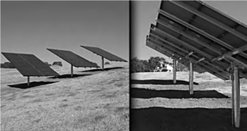
Figure B.5 Pipe-mounted semiadjustable tilt PV support structure.
