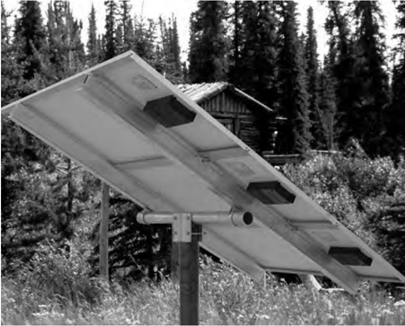
Figure B.8 Pipe-mounted semiadjustable tilt PV support structure.
