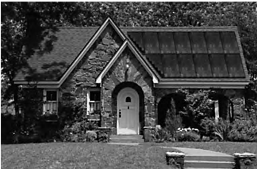
Figure B.28 Laminated glass solar power installation in residential building roof structure. Photo courtesy of Sharp Solar.
