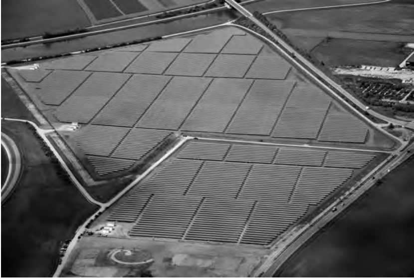
Figure B.32 10 single axis tracker Bavaria Solar Park. Photo courtesy of Sun Power.
