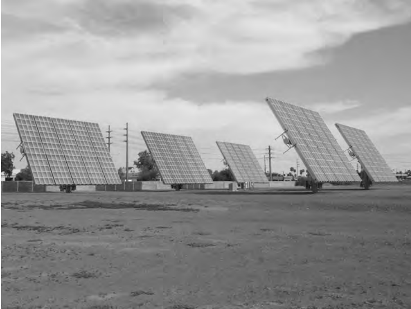
Figure B.21 25 KW Solar mega concentrator power co-generation farm. Photo courtesy of AMONIX.
