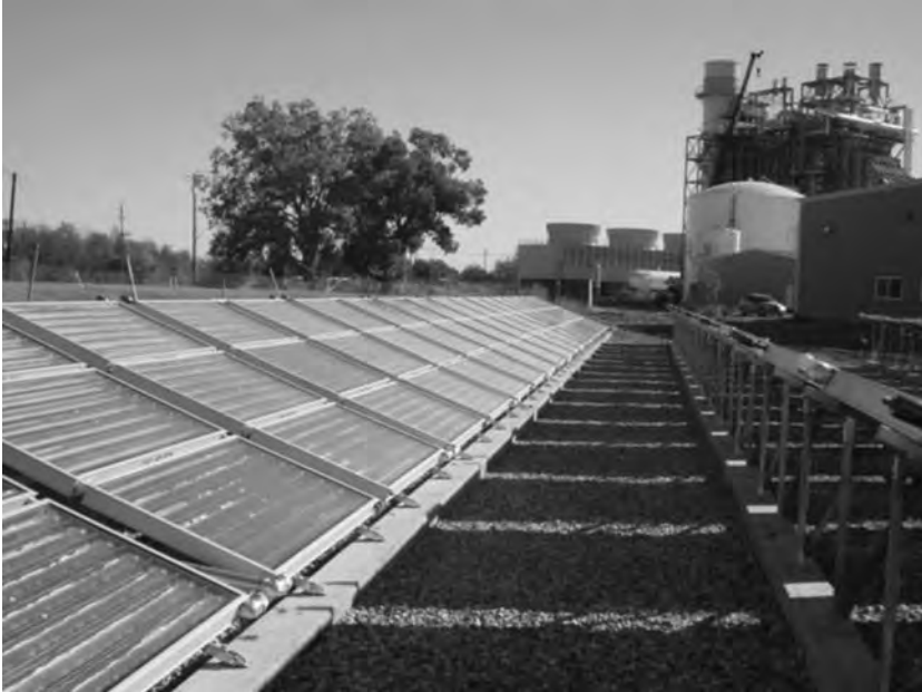
Figure 10.8 An industrial solar liquid heating panel installation.
