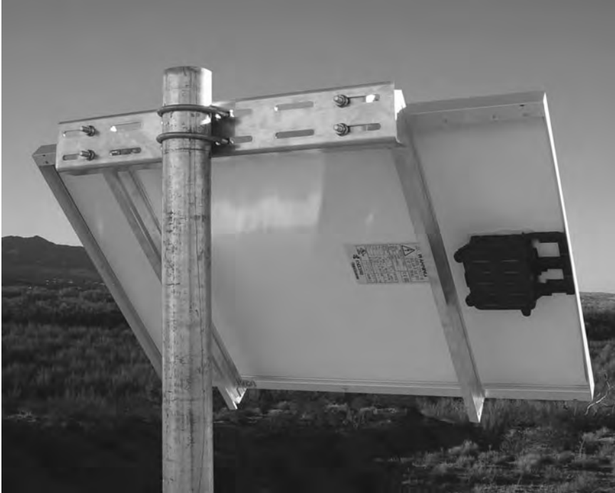
Figure 3.16 A single PV frame ground-mount solar power support.
